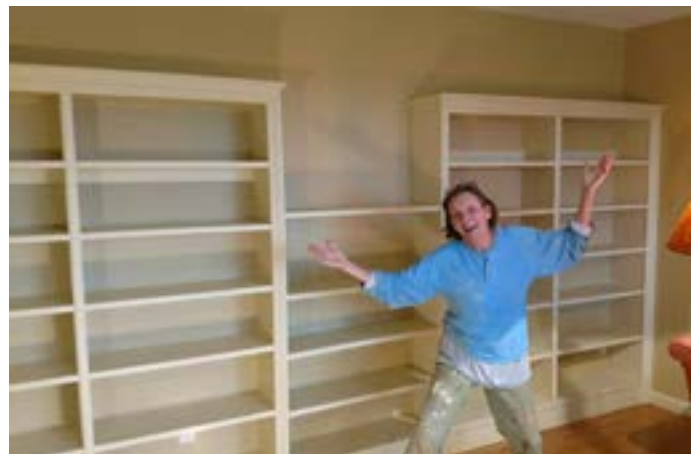
Gail having a ta-da! moment upon completing a set of built in shelves
